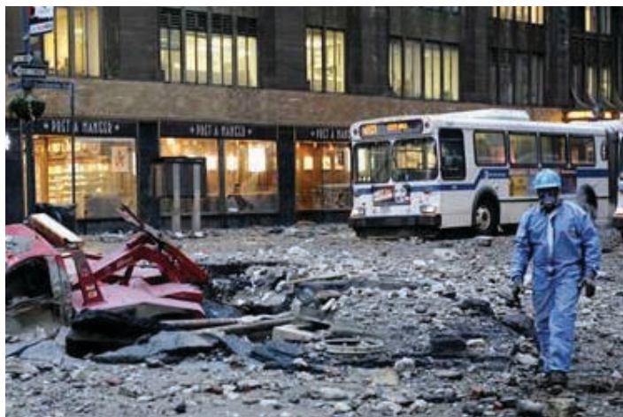
Water hammer caused devastation in New York.
