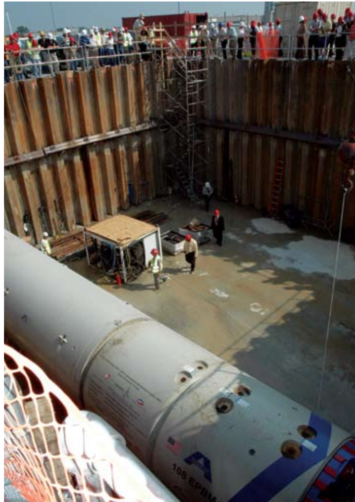
The Earth Pressure Balanced Tunneling Machine will drill a 2,016-foot, 9-foot diameter connector beneath a runway and two taxiways to house thermal and other utilities for the new Midfield Terminal.
