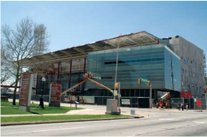
College campuses like IUPUI are responsible for considerable chilled water system growth world wide. The Campus Center will use steam and chilled water from Citizens Thermal Energy.
