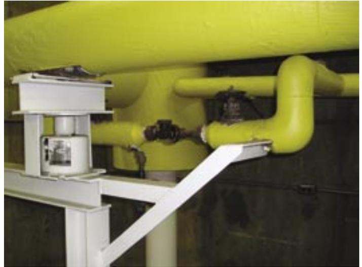
design) will malfunction. Ultrasonics, infrared temperature measurements and visual inspection have proven useful to maintenance personnel in checking for malfunctioning steam traps. Of the three, ultrasound is the most reliable. Visual inspection requires an inspector to let a steam trap discharge to atmosphere. However, doing that changes the parameters of the closed system and, therefore, can be unreliable.
