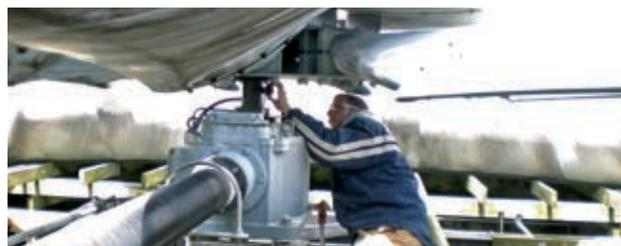
A Chilled Water Technician performs an alignment check on a cooling tower fan gearbox at the West St. chilled water facility.
