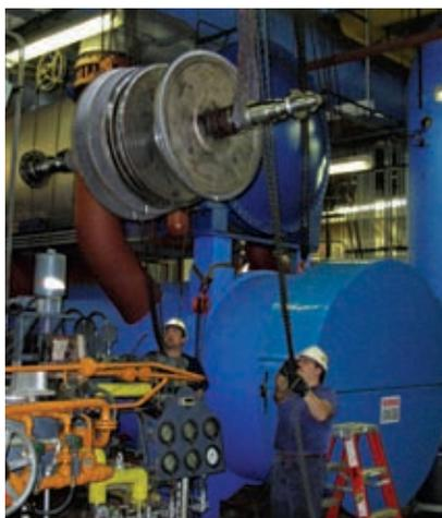
Chilled water maintenance personnel lower a re-conditioned steam turbine rotor back into place on one of the 5,000 ton steam driven chillers at the West St. chilled water facility.
