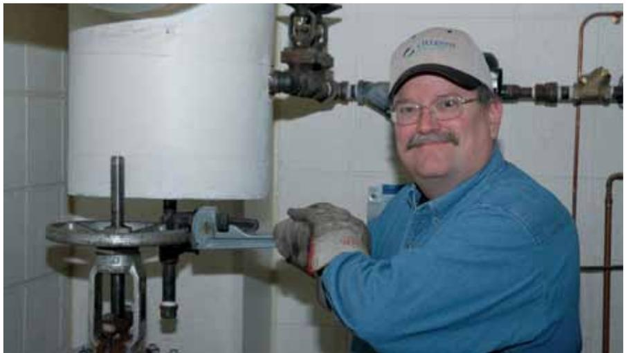
Citizens Thermal Industrial Steam Meter Man Jeff Sietsma shuts off the steam isolation valve at a customer's facility.
