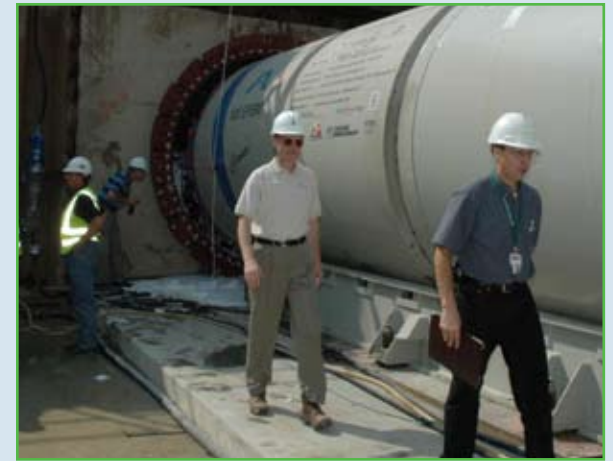
Citizens Thermal worked with a diverse group of contractors on the installation of the HVAC for the new Indianapolis Airport terminal.
